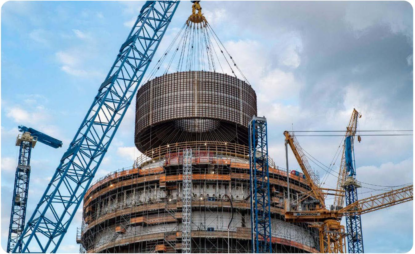
The CB-20 module being installed at Vogtle-3. Photo: Georgia Power
