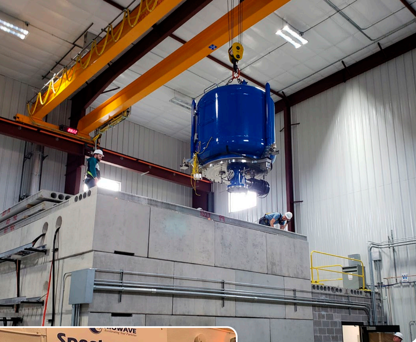
Above: A production component going up and over a bunker wall into a SHINE structure. Photo: Phoenix LLC
