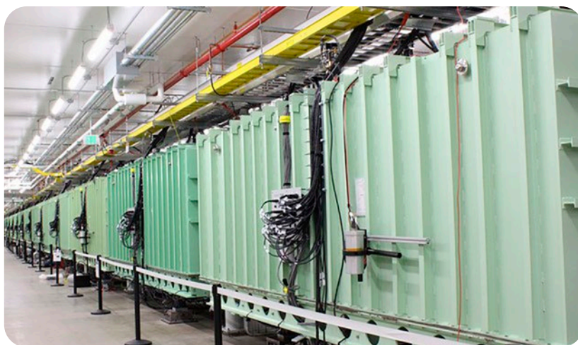
Superconducting magnets at the Facility for Rare Isotope Beams. Photo: FRIB
