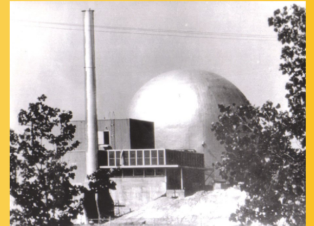
Piqua Nuclear Generating Station (1963) Organic cooled and moderated 45.5 MW th reactor
