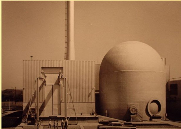
Pathfinder Nuclear Generating Station (1966) Superheated boiling water reactor 62.5 MW e reactor
