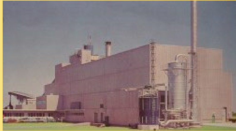
Hallam Nuclear Generating Station (1963) Liquid sodium and graphite moderated 75 MW e reactor
