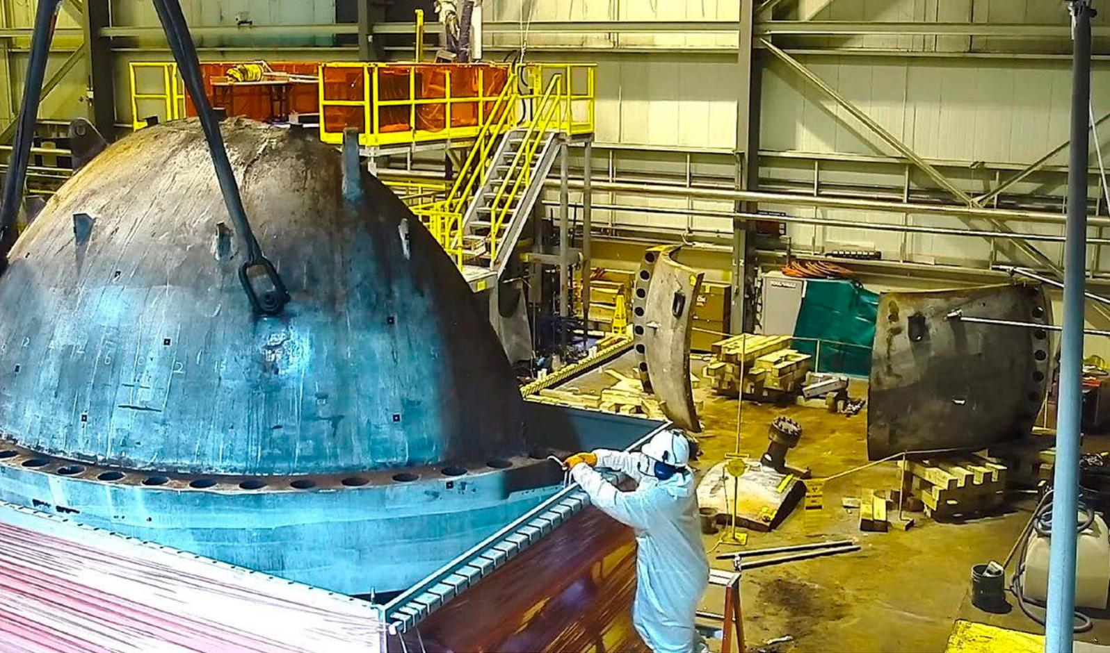
Vermont Yankee's segmented reactor vessel head is lowered into a custom-built package for transportation and disposal. (Photo: Orano)
