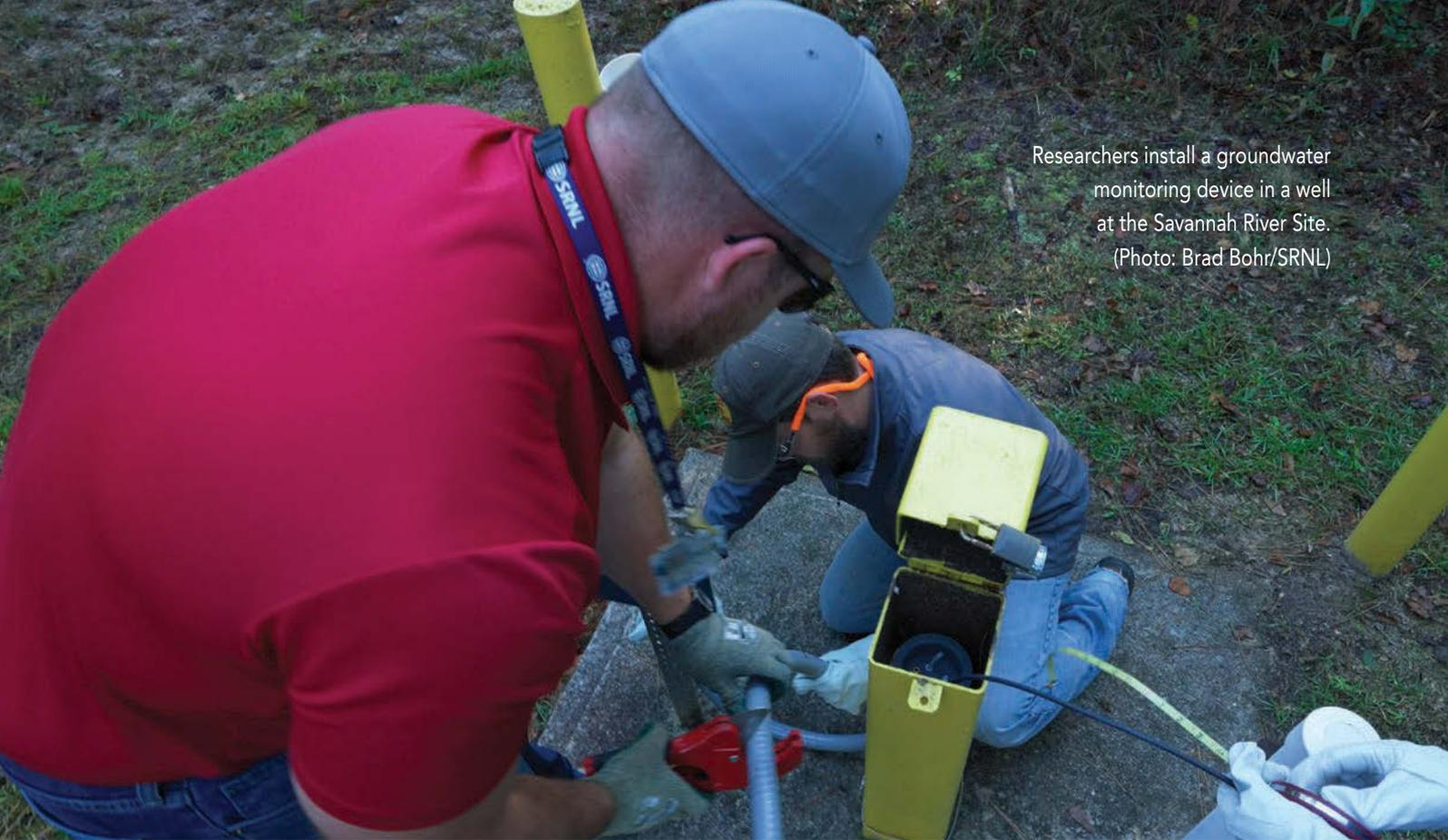
Researchers install a groundwater monitoring device in a well at the Savannah River Site. (Photo: Brad Bohr/SRNL)
