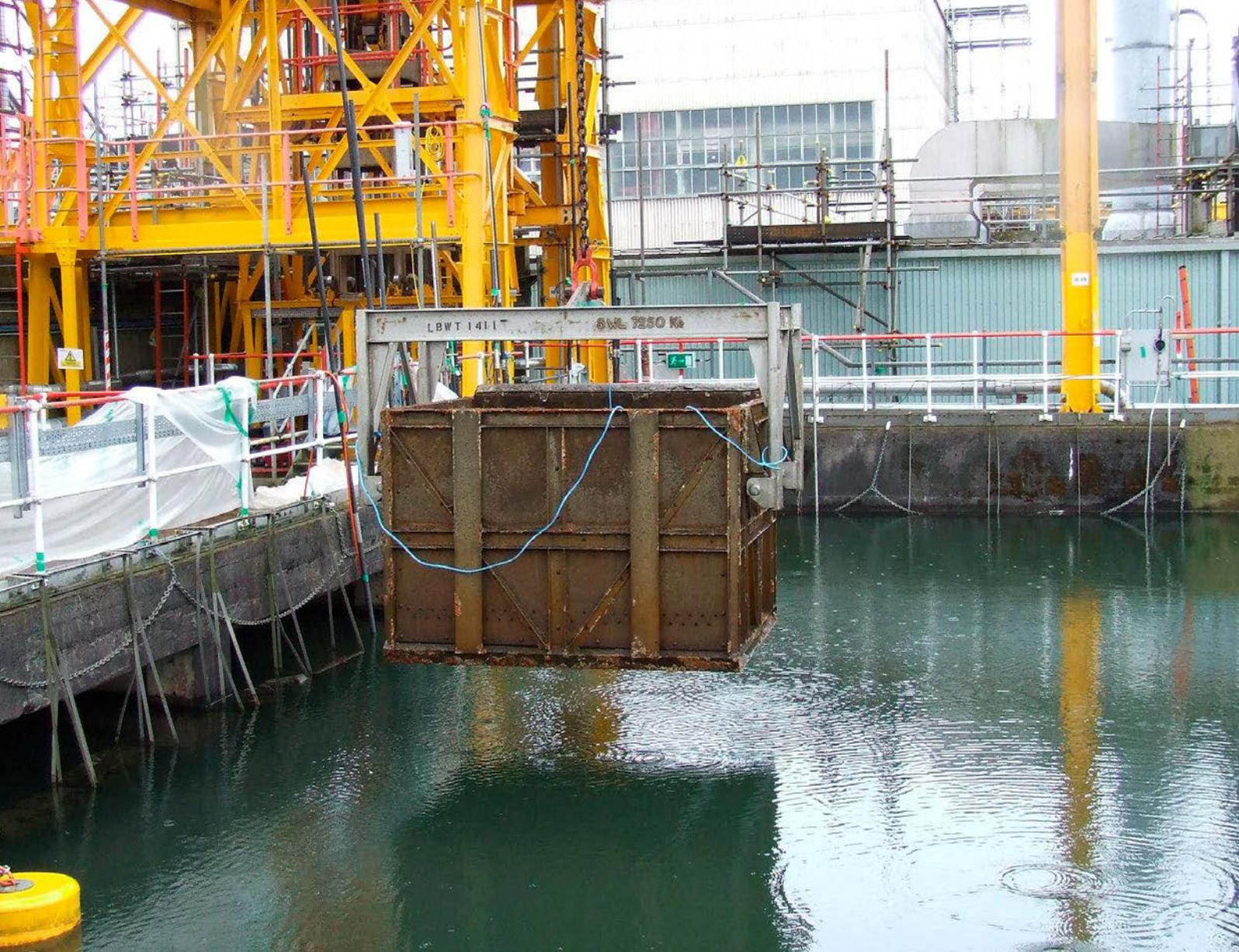
As part of an earlier campaign to remove intermediate-level waste, a fuel skip is removed from the storage pond. The facility was placed into a passive care and maintenance regime in the 1970s, until a remediation program was initiated in the 1990s.
