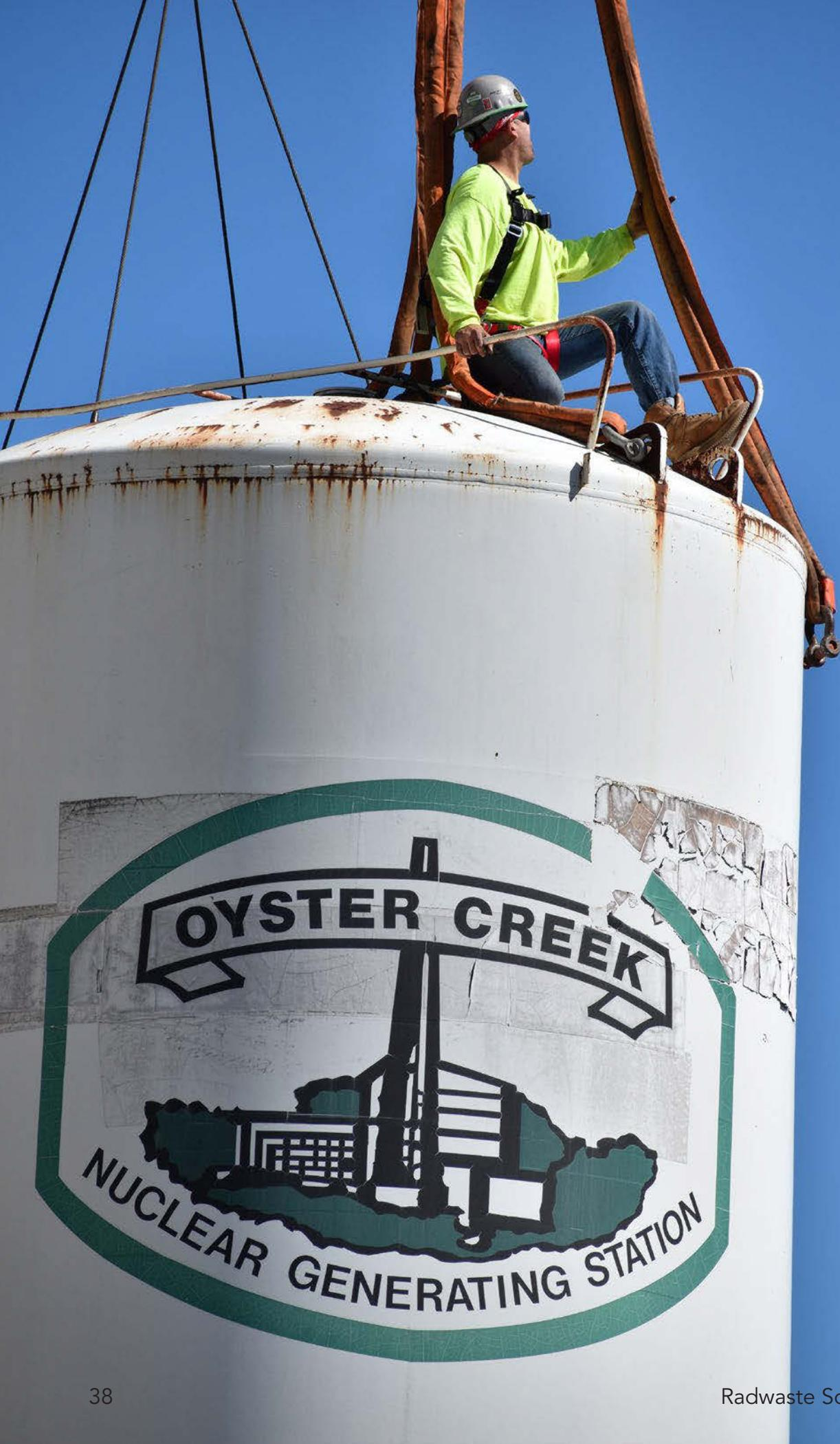
A rigger prepares a nitrogen storage tank to be taken down at the Oyster Creek nuclear power plant in New Jersey. (Photo: HDI)
