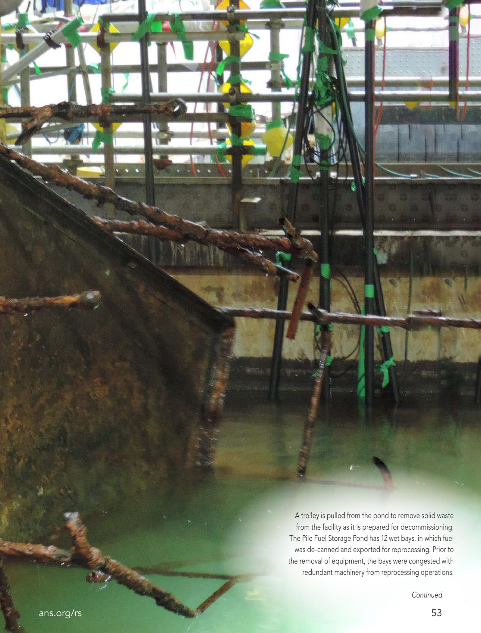
A trolley is pulled from the pond to remove solid waste from the facility as it is prepared for decommissioning. The Pile Fuel Storage Pond has 12 wet bays, in which fuel was de-canned and exported for reprocessing. Prior to the removal of equipment, the bays were congested with redundant machinery from reprocessing operations.
