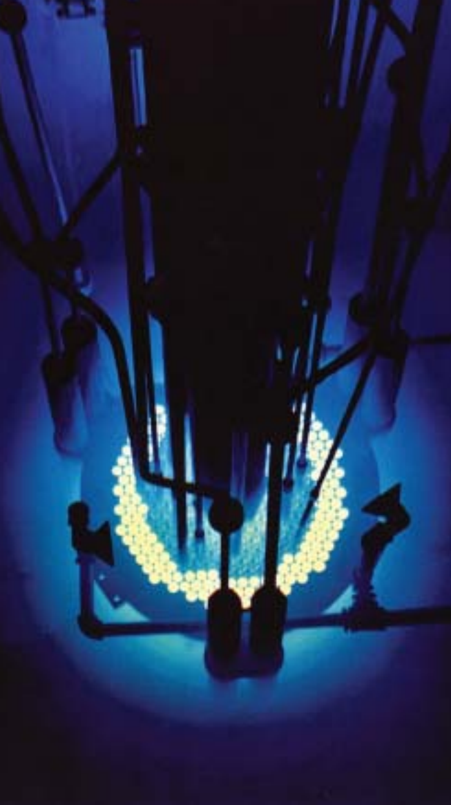
Fig. 17. Dry central cavity in annular core pulsing reactor
