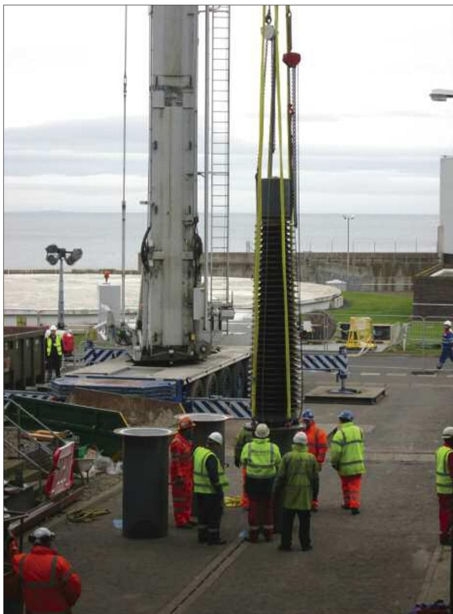
Torness-1’s transformer bushings are lowered to the ground outside the Unit 1 reactor building.
