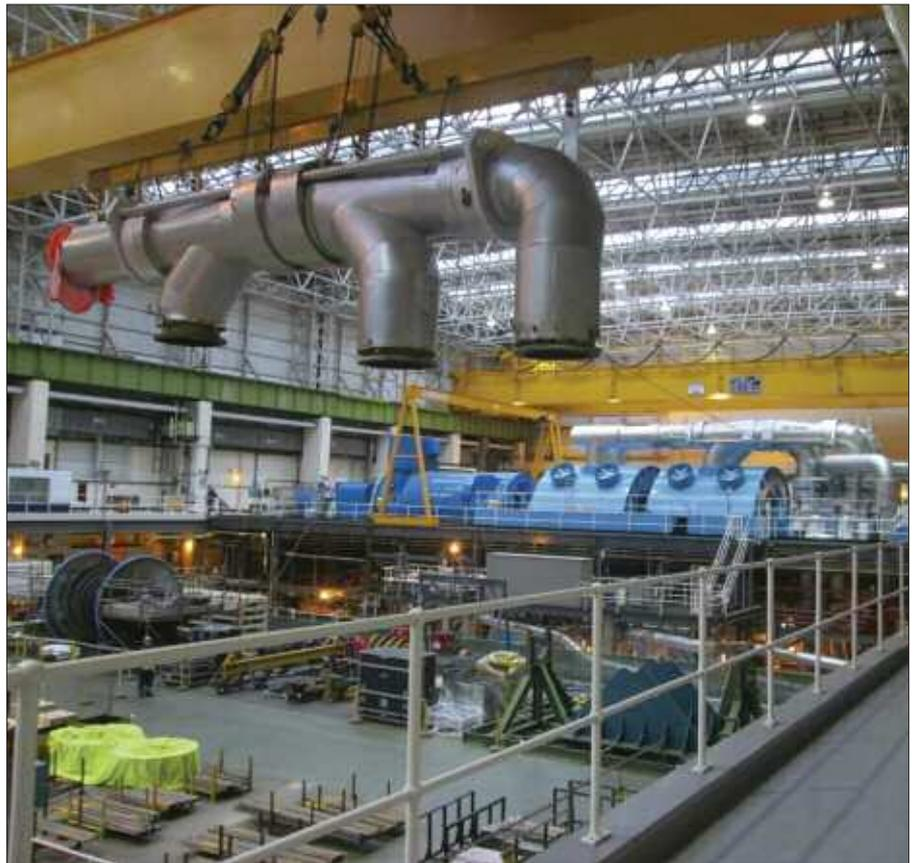
The 30-metric-ton low-pressure steam crossover pipe is removed from the Torness-I turbine.
