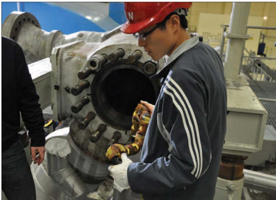
CMU mechanical engineering Ph.D. student Chaohui Gong deploys the Biorobotics Lab's snake robot into the Zwentendorf nuclear power plant's turbine room steam piping through a spherical vessel.
