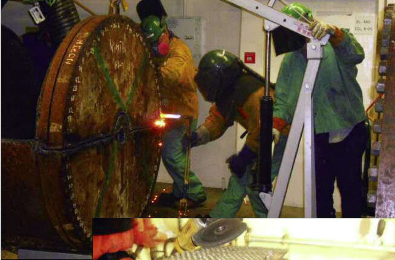
**Above:** Work in the auxiliary building includes the segmentation and size reduction of equipment for disposal as Class A low-level waste.
