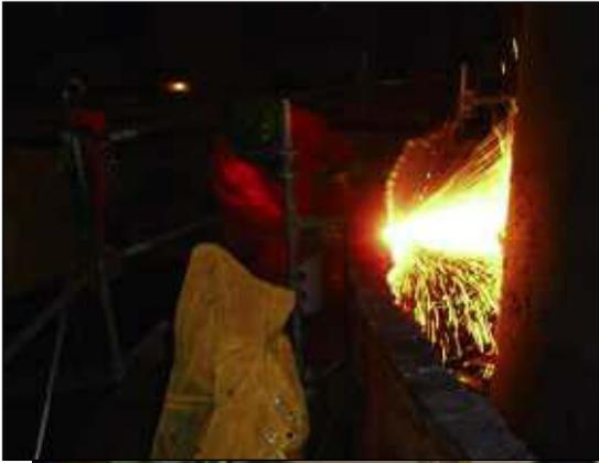
**Left:** The upper portions of the Unit 1 steam generators are segmented in place to facilitate the future removal of the lower portions. The upper portions were packaged and loaded into railcars for transport to and disposal at EnergySolutions' low-level waste disposal facility located in Clive, Utah.
