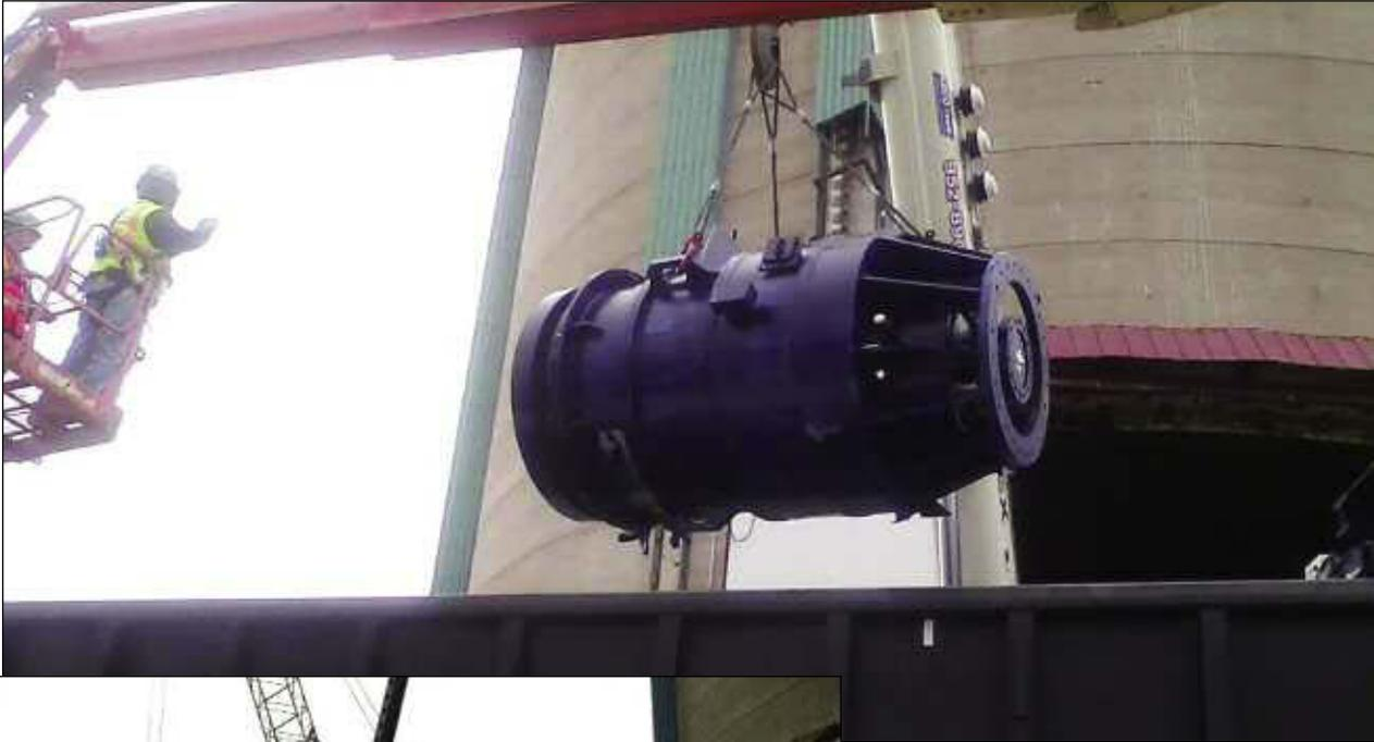
**Opposite page, top:** Waste from the Unit 2 containment is placed into a railcar using the heavy-lift rail system and crane.
