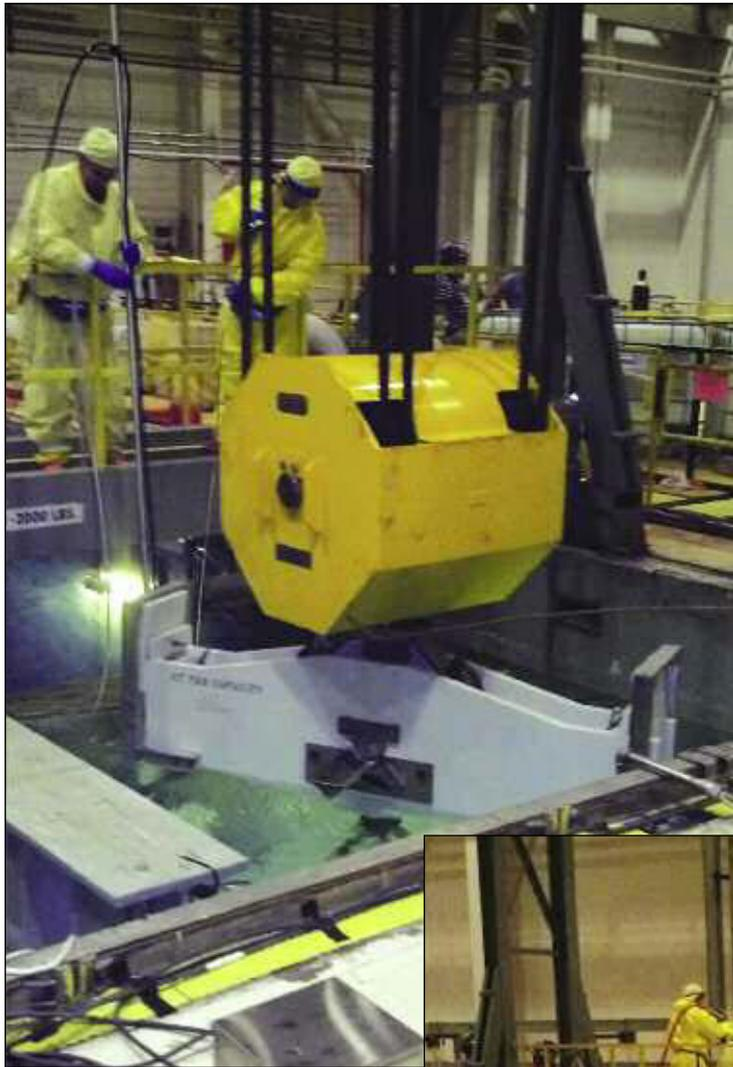
**Left:** The fuel transfer cask is lowered into the spent fuel pool using the fuel building's crane.
