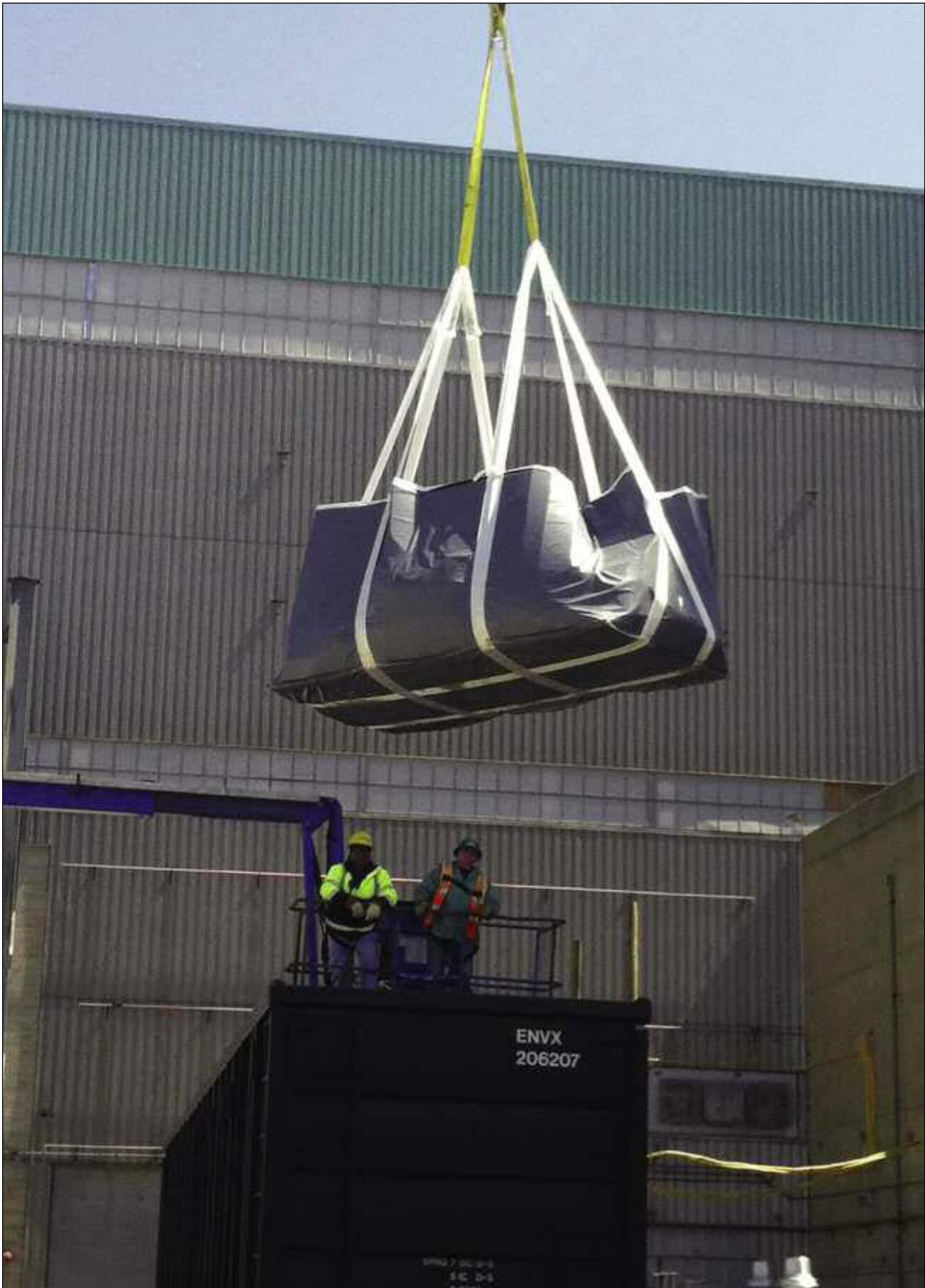
*Class A waste material being removed from the auxiliary building is packaged first into sacks, as shown, to facilitate loading into railcars while also controlling potential contamination.*
