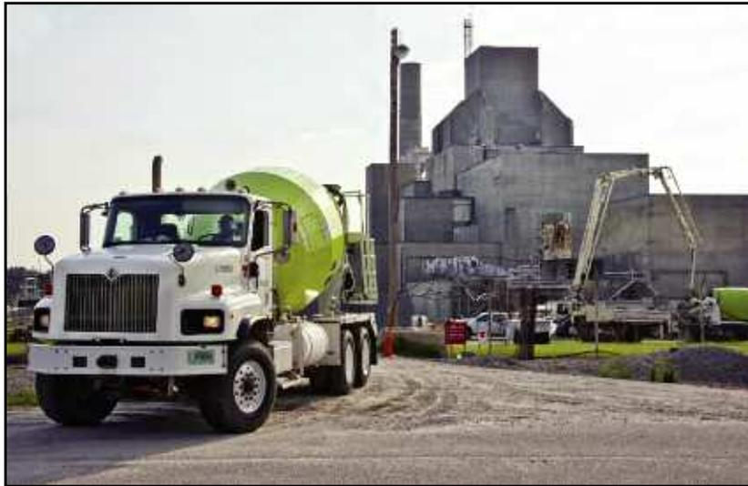
More than 2.8 million gallons of cement-like grout were recently poured into SRS's dormant C Reactor facility to safely eliminate a potential source of contamination while fully preserving the historical integrity of the building.
