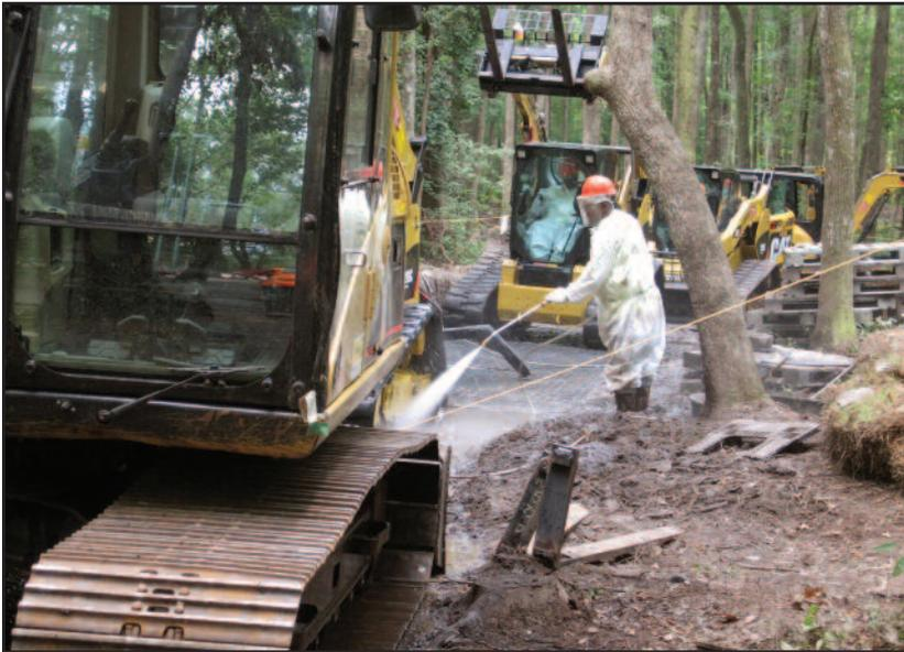
Power washers ensured the removal of any radioactive contamination clinging to heavy equipment used to remove soil near Lower Three Runs at SRS. The equipment was then radiologically surveyed to confirm acceptable release limits were met.
