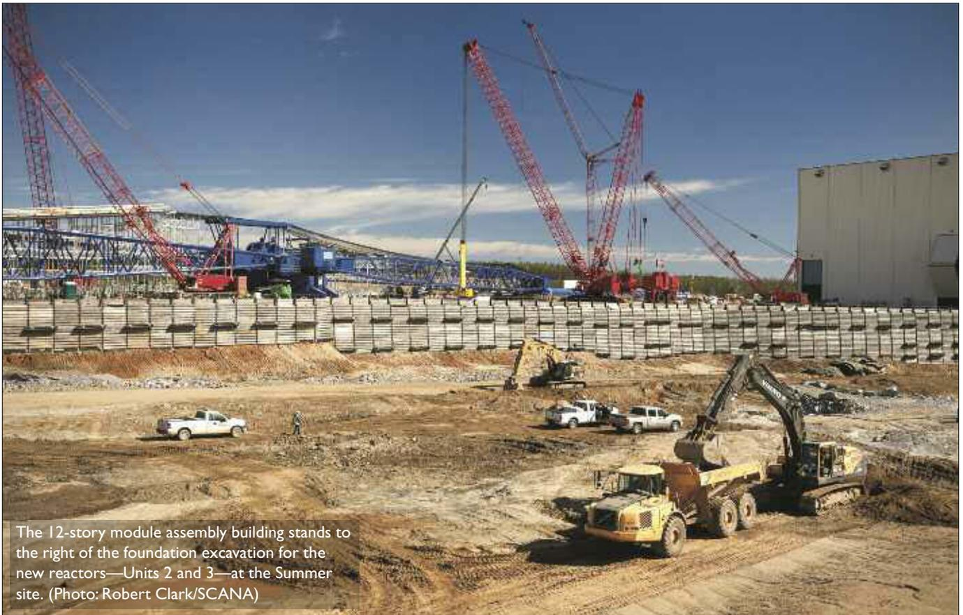
The 12-story module assembly building stands to the right of the foundation excavation for the new reactors—Units 2 and 3—at the Summer site. (Photo: Robert Clark/SCANA)
