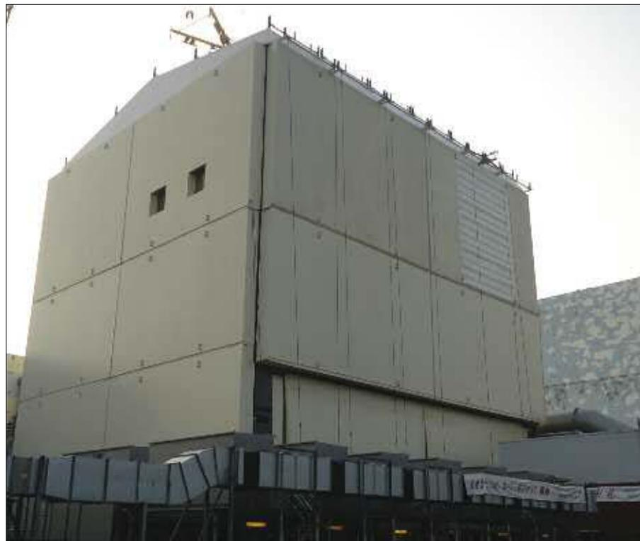
. . . and on October 14, 2011, nearing the completion of the unit's new outer structure, which is designed to contain airborne contamination (Photos: Tepco)
