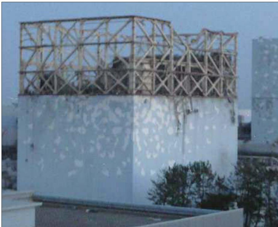
Unit 1 at the Fukushima Daiichi nuclear power station on March 12, 2011, following the earthquake and tsunami and after an explosion that opened up the top of the outer reactor building's shell . . .
