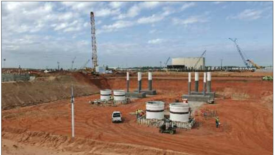
This shot of the Vogtle new construction site, taken on November 3, 2011, shows circulating water system pipes that will connect to Unit 3's turbine building and condenser. (Photo: Southern Company)
