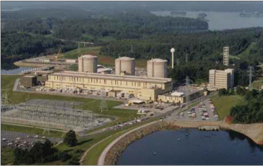
The I&C upgrade has been finished at Oconee's Unit 1 (left). Unit 3 (right) will be upgraded in 2012, and Unit 2 (center) in 2013.
