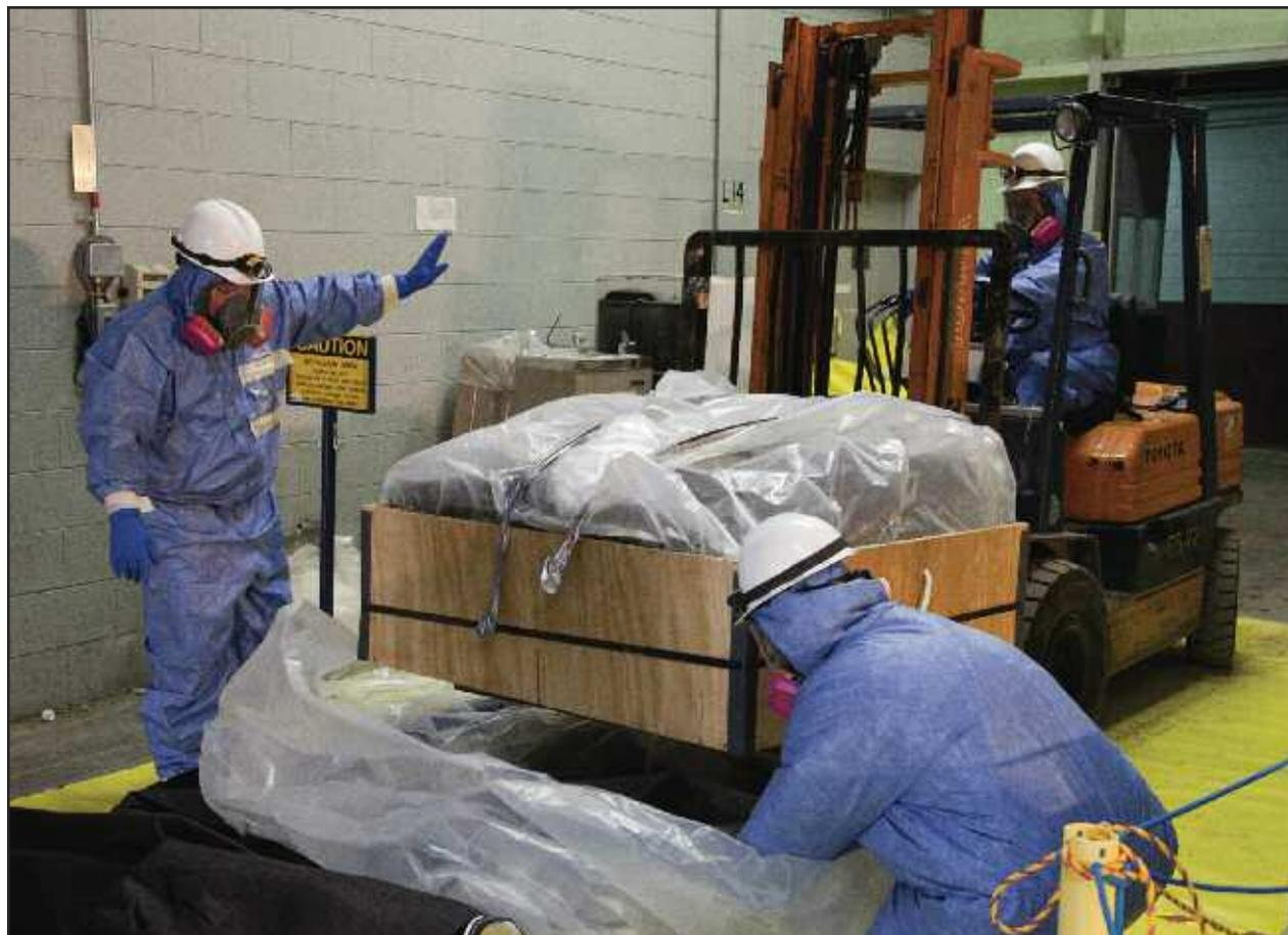
*Loaded and inspected plywood box being lowered into super-sack for shipment offsite.*
