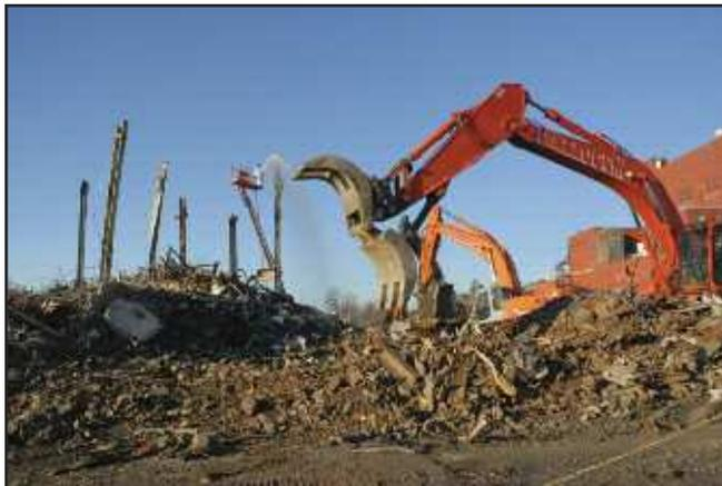
*Building 9211 D&D almost complete, with excavator removing rubble from building site.*
