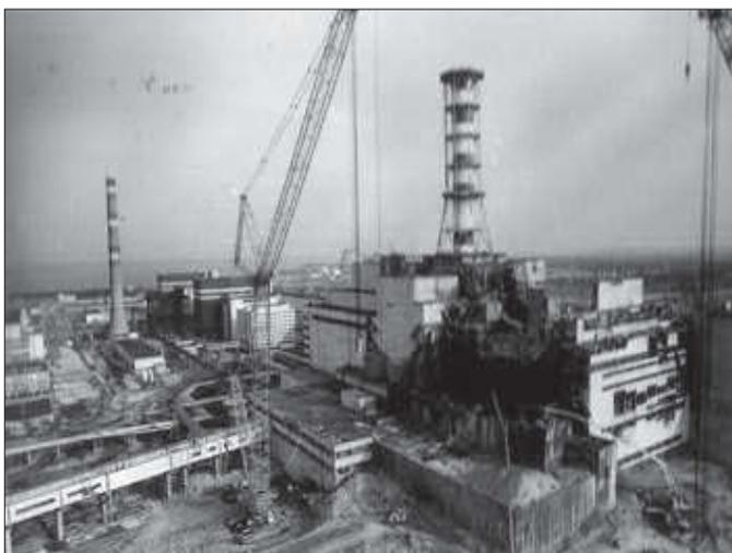
A 1986 aerial view of the destroyed Unit 4 at Chernobyl (left), and the start of construction of the original sarcophagus
