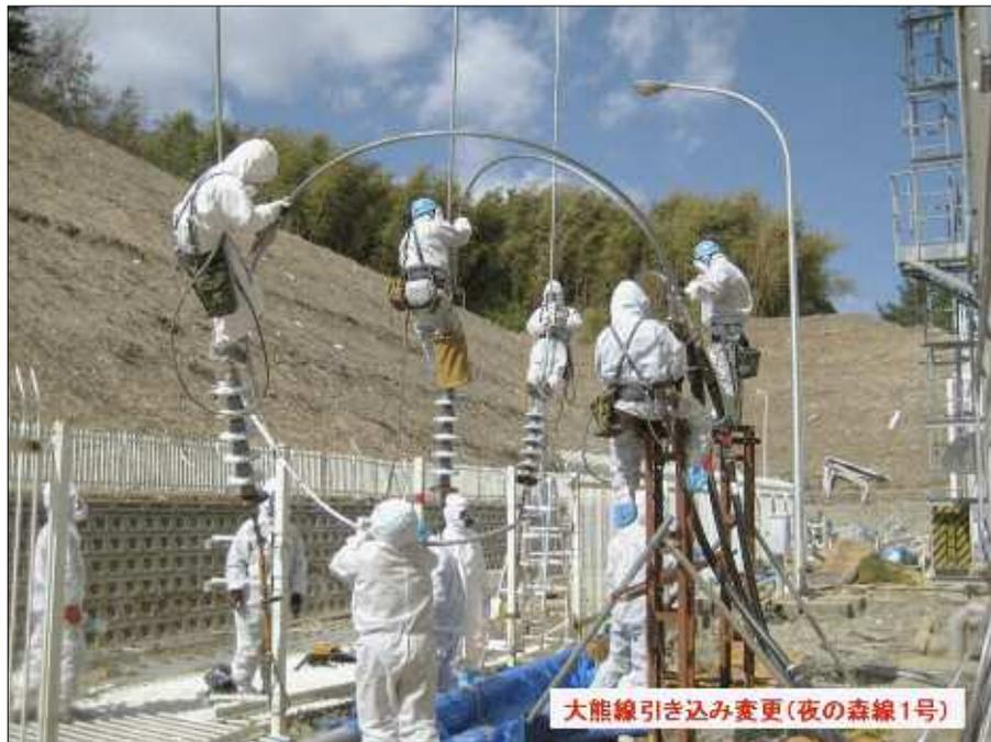
On March 18, workers repair equipment in an effort to restore off-site power to Units 3 and 4 at Fukushima Daiichi. (Photo: Tokyo Electric Power Company/Kyodo via AP Images)
