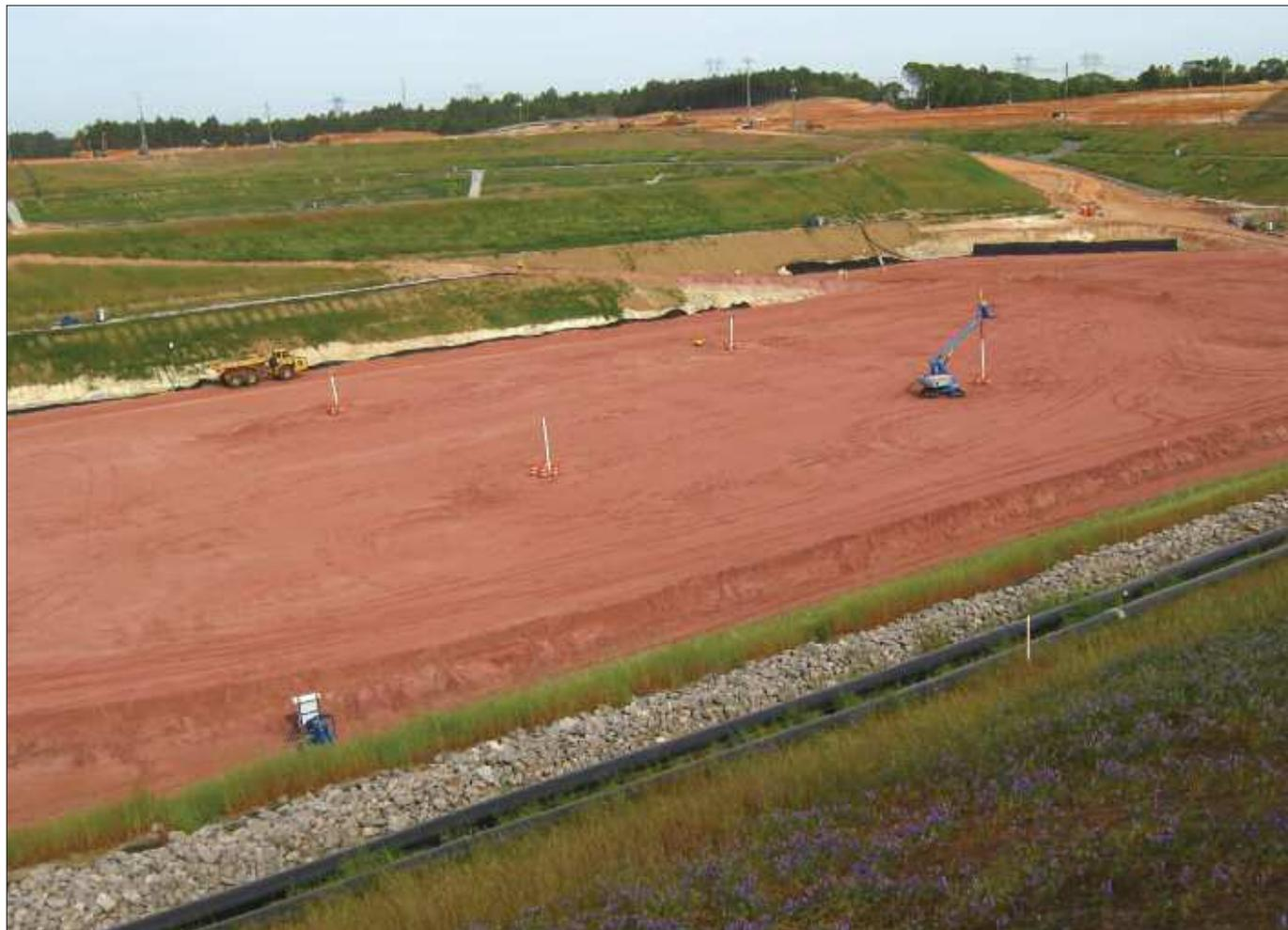
The Vogtle-3 excavation contained about 8 feet of backfill at the time of this photo (April 19). The slopes surrounding the excavation are terraced every 30 feet of height, with ramps to allow equipment to enter and leave.
