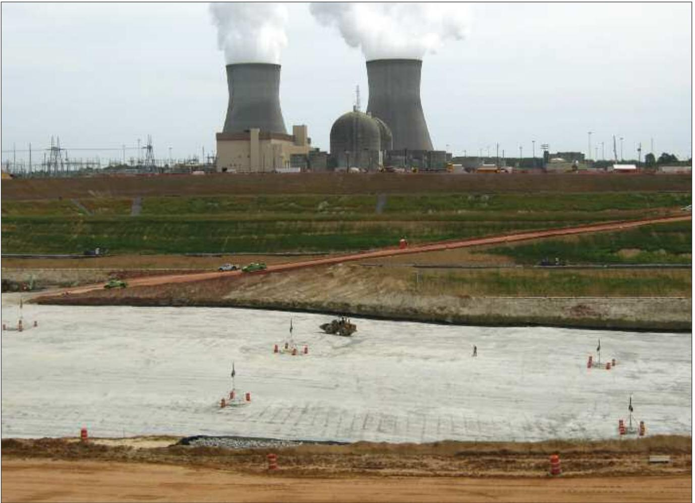
On April 19, backfilling had not yet begun for Vogtle-4. The structures on the blue bluff marl measure the vertical motion of the rock; with the 90-foot depth of dirt removed, the marl had risen measurably, and it was expected to lower again once the backfill was placed. Units 1 and 2, both in operation at the time, are in the background.
