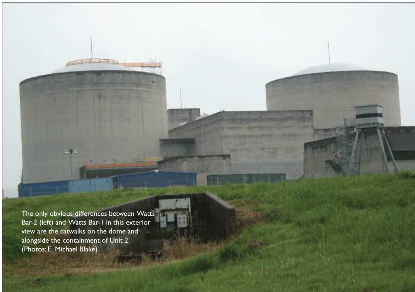
The only obvious differences between Watts Bar-2 (left) and Watts Bar-1 in this exterior view are the catwalks on the dome and alongside the containment of Unit 2.
