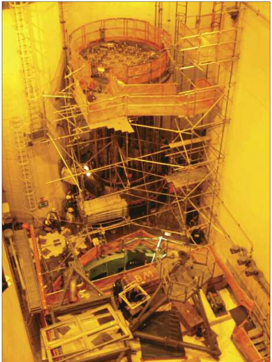
Inside the Watts Bar-2 containment, work proceeds simultaneously in several areas, in close quarters. The reactor vessel upper head, with control rod drive tubes in place above it, is shown in the background, surrounded by scaffolding. In the foreground, partly obscured, is the open cylinder of the reactor vessel.
