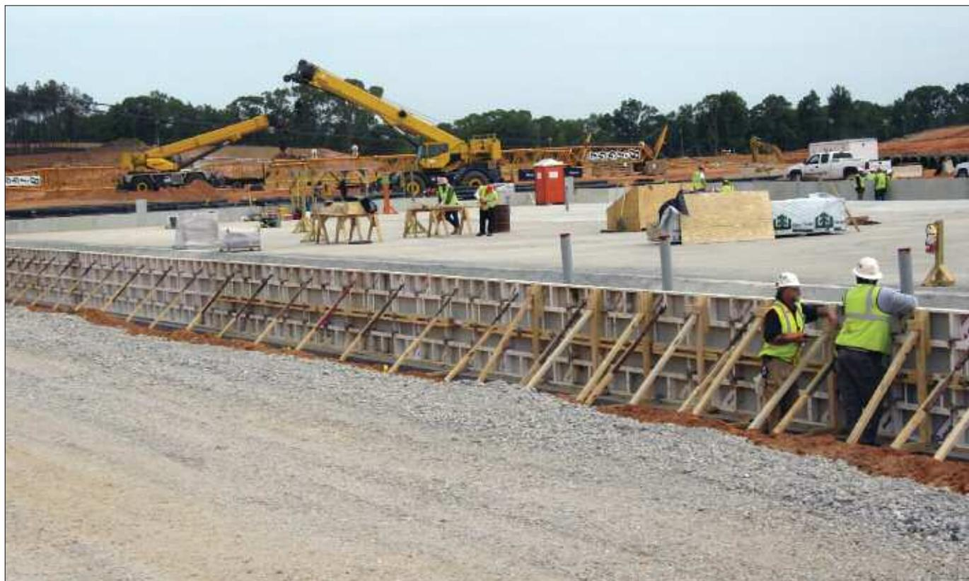
The foundation has been completed for the module assembly facility at Vogtle. Work on the building's other structures was just beginning.
