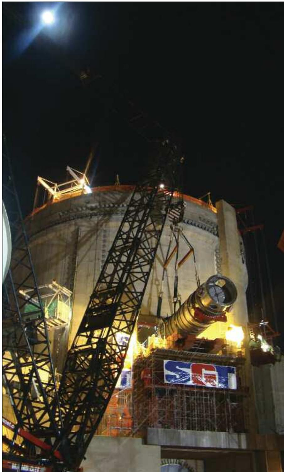
Under a full moon, a new steam generator is moved inside of the reactor building.
