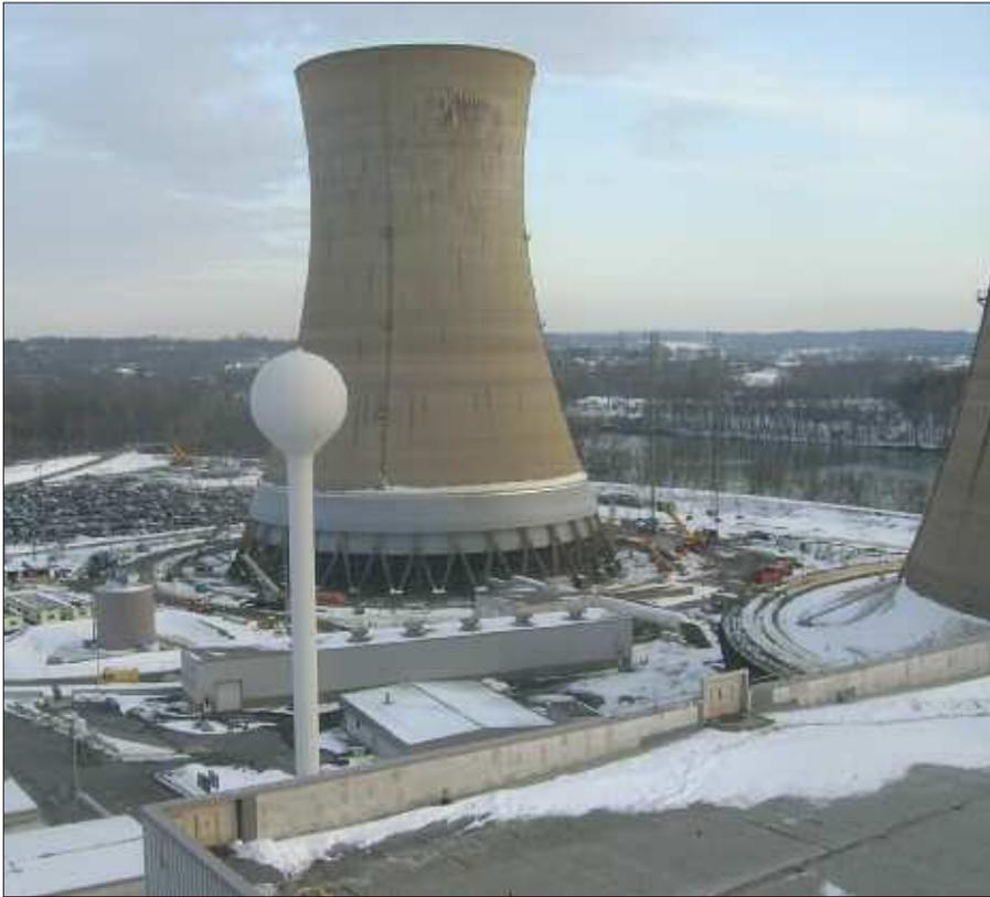
The drift eliminator on TMI-I's "A" cooling tower, which extended out about 30 feet all the way around the base of the tower, was removed during the outage. The plant's "B" cooling tower, of which part of the base can be seen at right in the photo, still has its drift eliminator in place.
