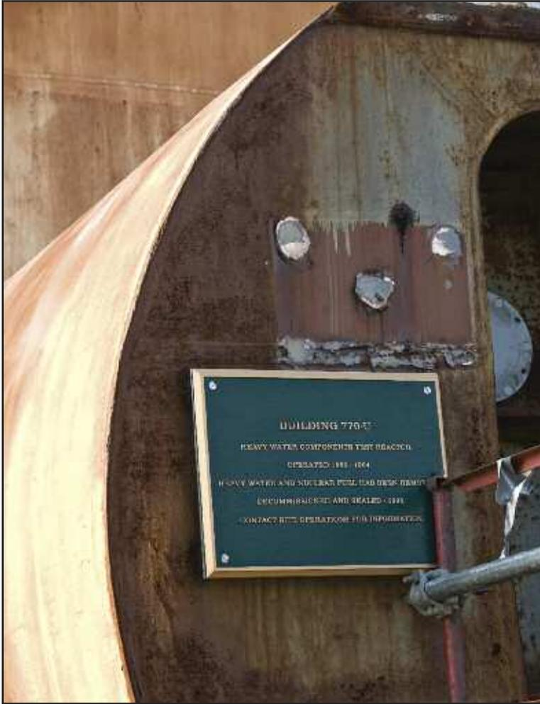
*The HWCTR ran from 1961 to 1964 and has been welded shut since 1998.*
