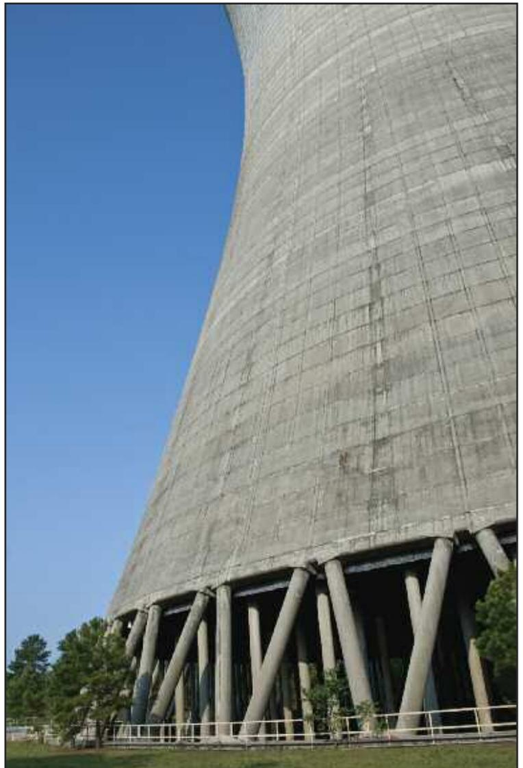
*The 450-ft K Area cooling tower is built on concrete stilts and has a water-filled basin underneath*
