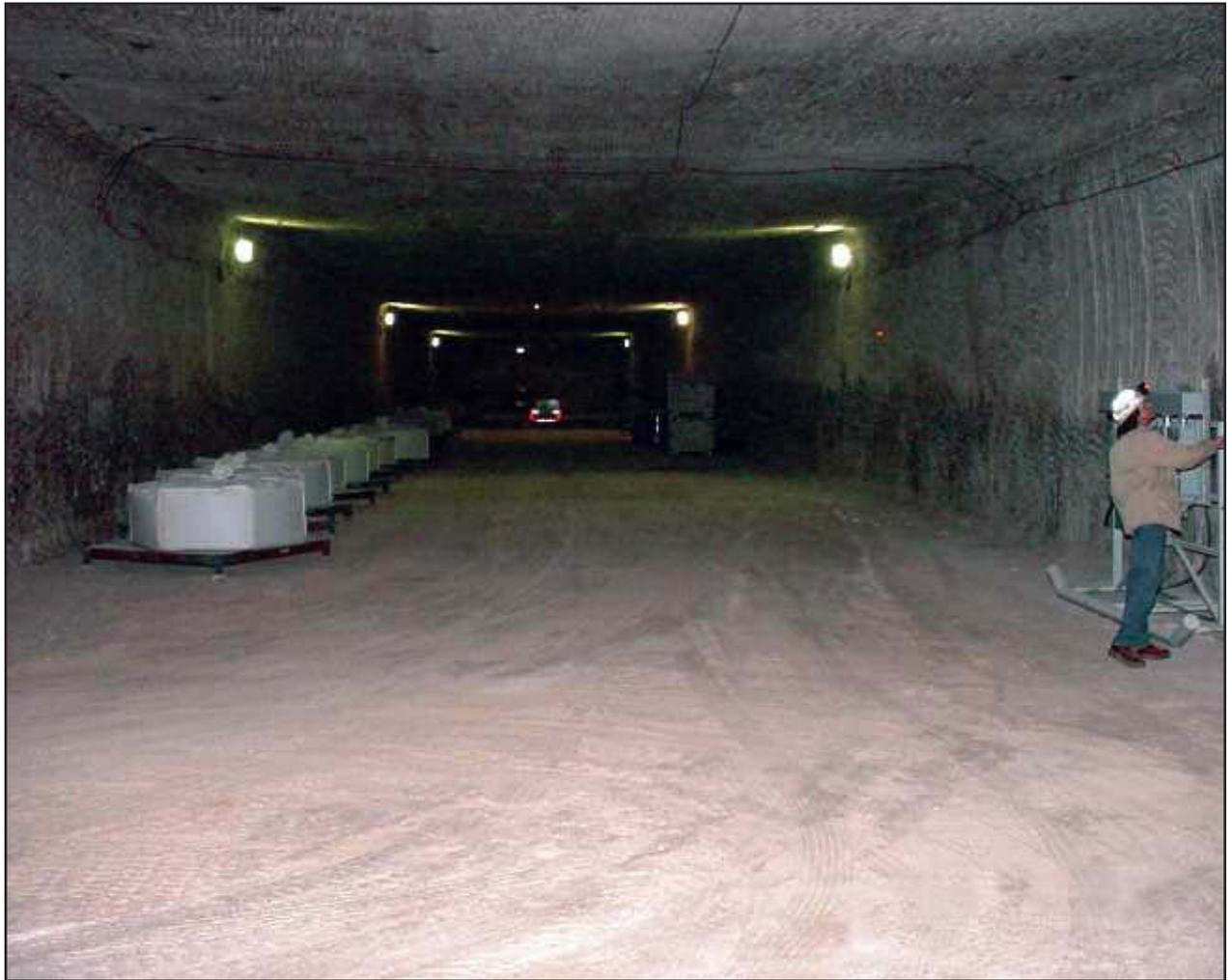
*A newly ready disposal room in Panel 3 showing width and height before significant closure begins. Note the comparative lack of roof bolts.*
