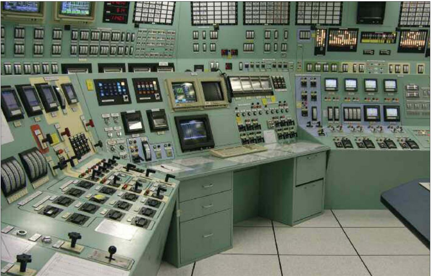
A conventional analog control room in a nuclear power plant (Photo: NRC)
