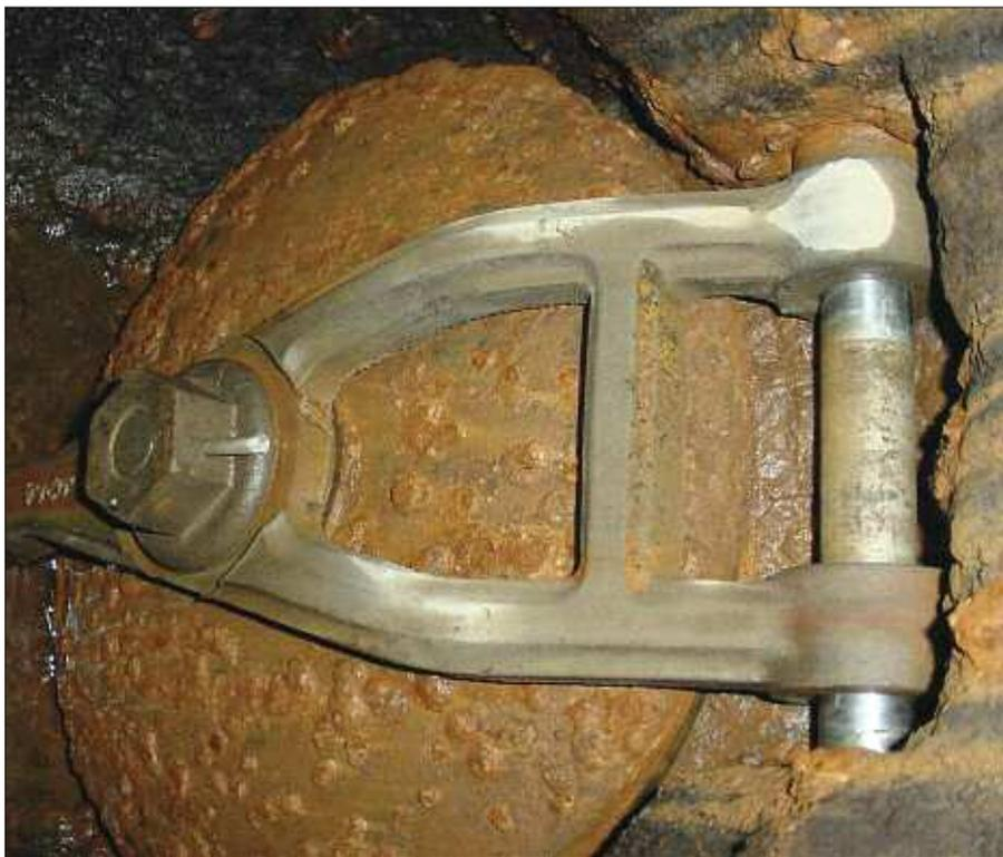
A check valve with improved material used on the hinge and fasteners
