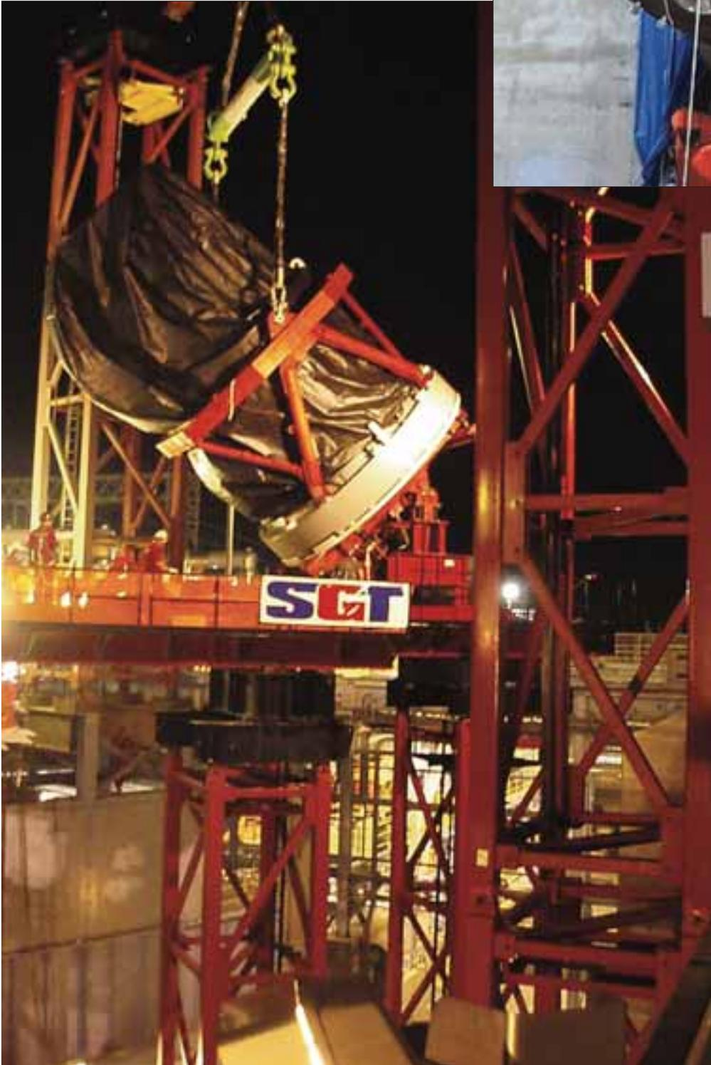
■ The binding and the uncentered position of the cooling water system block on a temporary lifting device.
