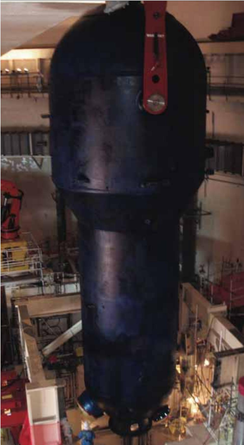
An original steam generator is removed from its cubicle inside the containment building. Both of the original steam generators were treated with a blue anticontamination coating prior to their removal. They were to be shipped to a disposal facility in Memphis, Tenn.
