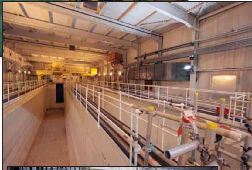
contamination is in the areas that had been submerged in pond water. Following the draining of the ponds in 1997, sampling indicated that approximately 40 mm of surface material had to be removed. This measurement equates to a total of approximately 300 tonnes of concrete and embedded steel items that had become contaminated during the operational life of the station
