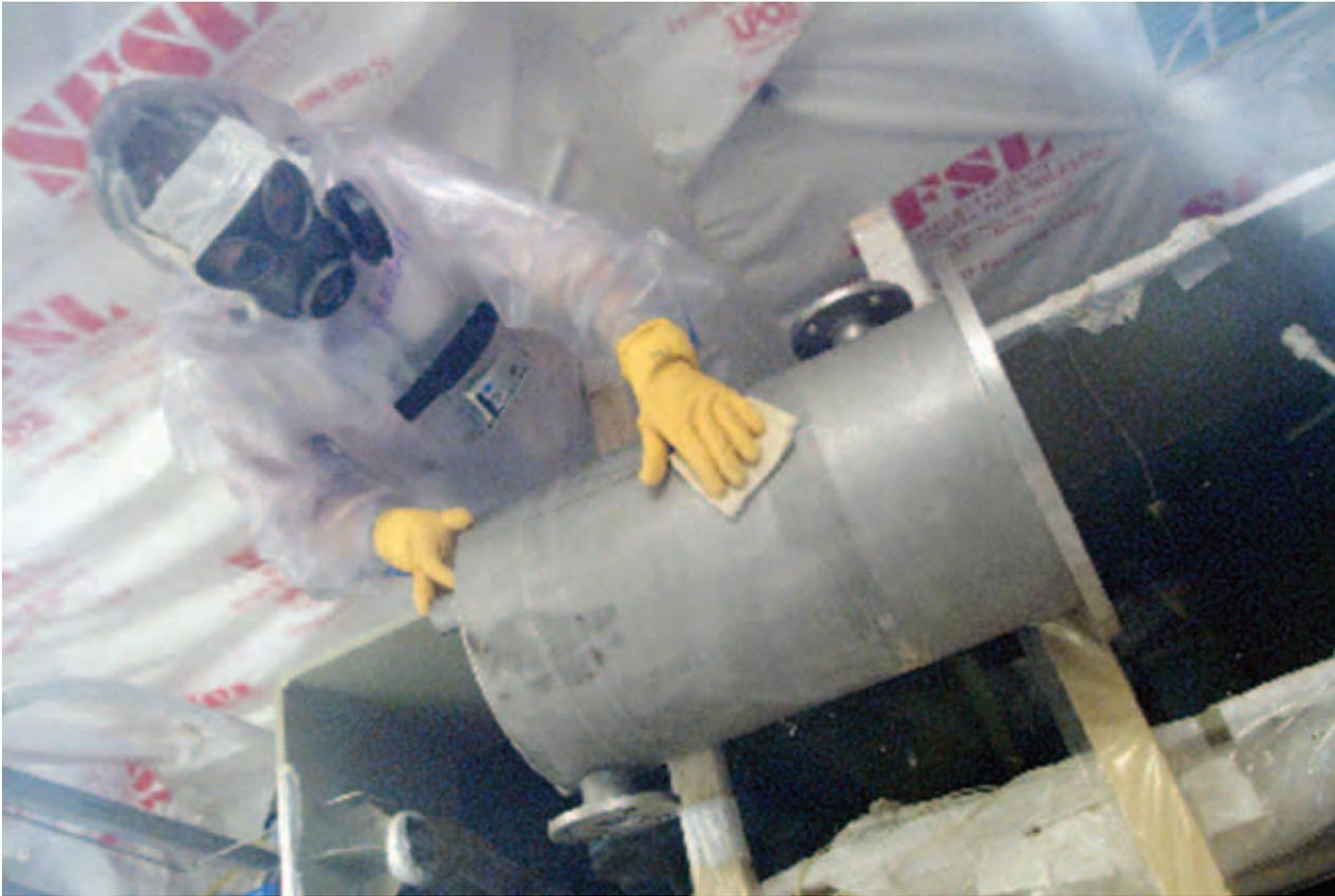
Fig. 3. Filter housing decontaminated to background radiation levels.
