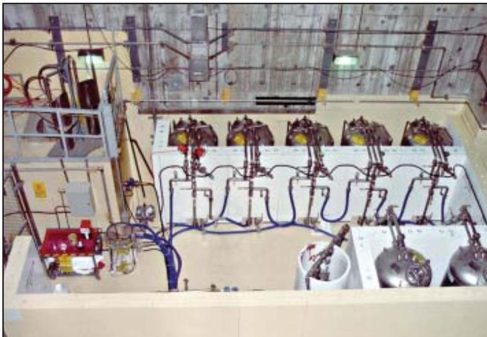
Fig. 2. Typical in-service filtration demineralizer system.
