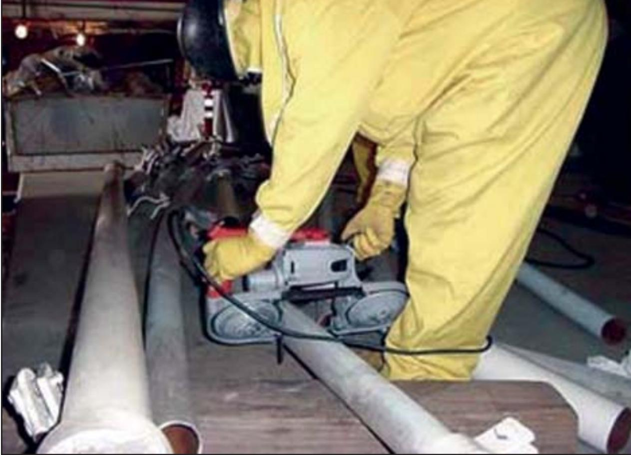
*Cutting pipe using a band saw (launderable protective clothing).*
