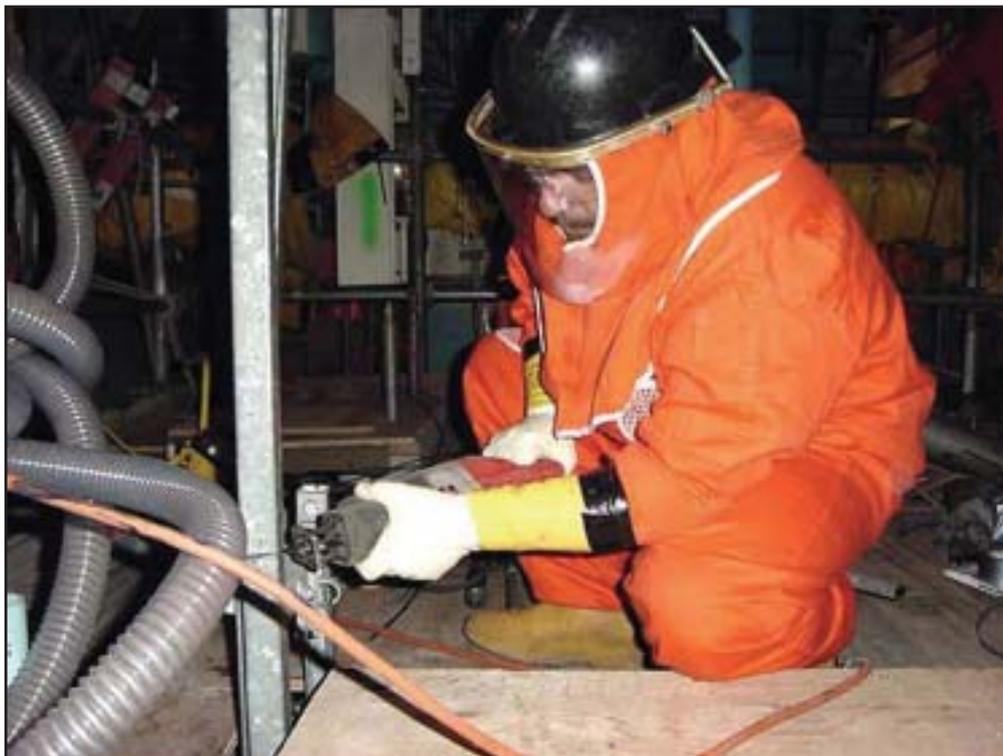
*Cutting pieces of Unistrut using a reciprocating saw (nonflammable clothing).*
