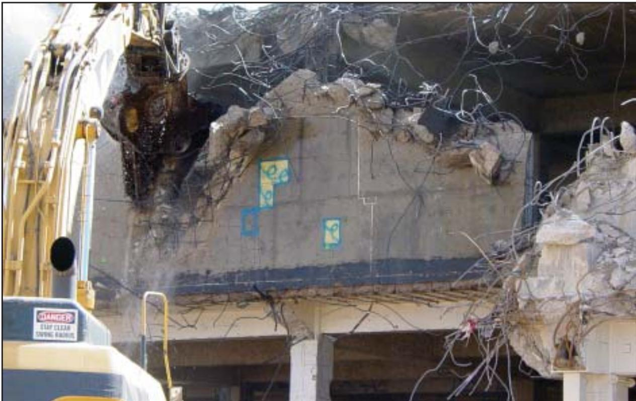
Spots of contamination from Building 771 structural concrete are sealed with an encapsulant and marked in bright colors. This allows demolition workers to easily identify pieces of concrete that will be packaged for low-level radioactive waste disposal. The remainder of the building, once called "the most dangerous building in America" by ABC News' *Nightline*, was decontaminated to free-release levels.
