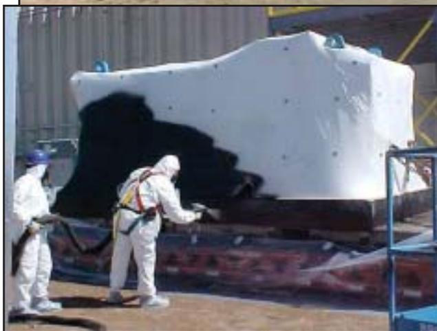
Rather than manually size-reducing large pieces of contaminated equipment to fit into approved waste containers, Kaiser-Hill worked with a vendor to develop a polyurea spray-on coating that served as the U.S. Department of Transportation-approved waste packaging for transportation. The innovation resulted in significantly reduced worker exposure to hazards. The largest item shipped from Rocky Flats was a 150-ton Sutton press (above).
