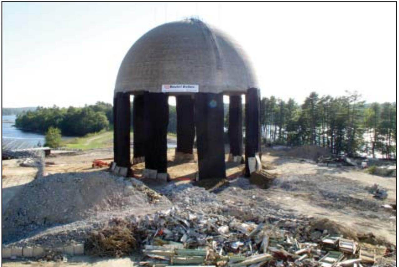
Eerily reminiscent of ancient temple ruins, the containment stands ready for the explosion, with the columns wrapped in fabric and chain-link fencing to minimize flying debris.
