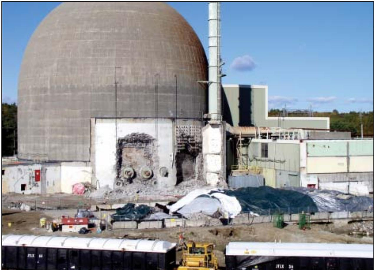
Areas where concrete and steel will be removed to create arches are outlined on the Maine Yankee containment building.
