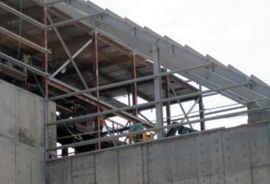
*D Reactor roof frame shows how new steel was joined to old steel so workers can apply galvalum roof panels.*
