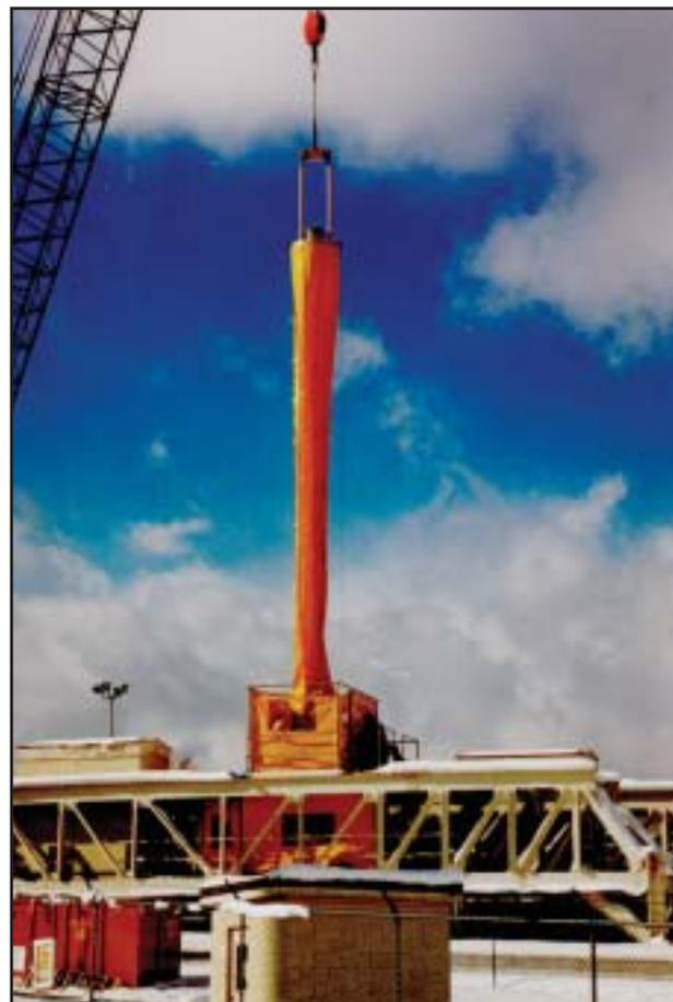
*Waste pumps that were removed from HLW tanks will be size-reduced and packaged in the remote facility.*
