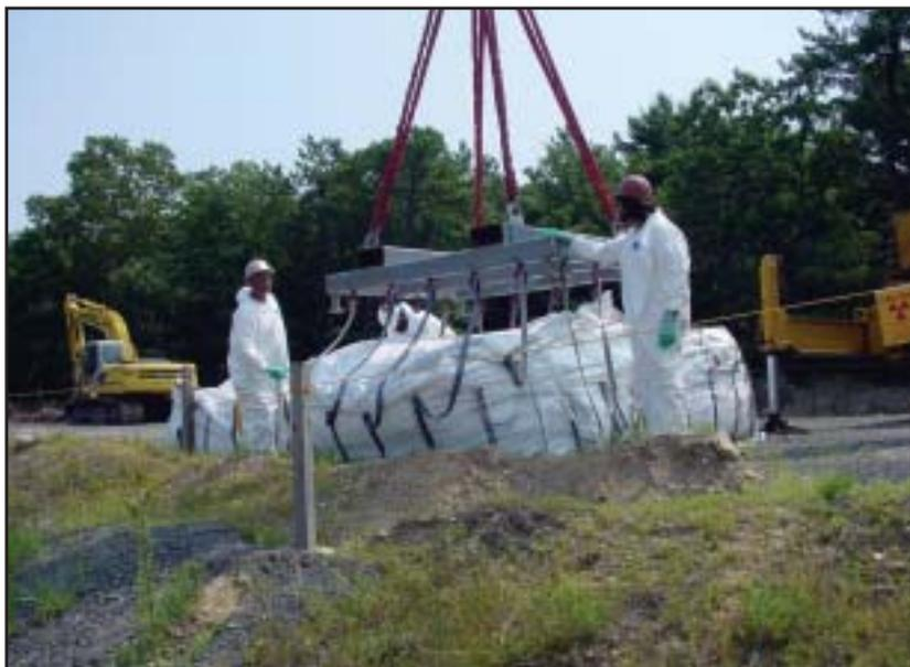
Workers attaching lifting straps to lifting frame to raise MHF Logistical Solutions flexible Lift Liner, which can carry up to 24 000 lb of radioactive materials. Location: Brookhaven National Laboratory, Long Island, N.Y.
