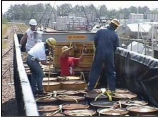
*Drums of depleted uranium oxide from the SRS being loaded in an MHF Logistical Solutions gondola railcar.*
