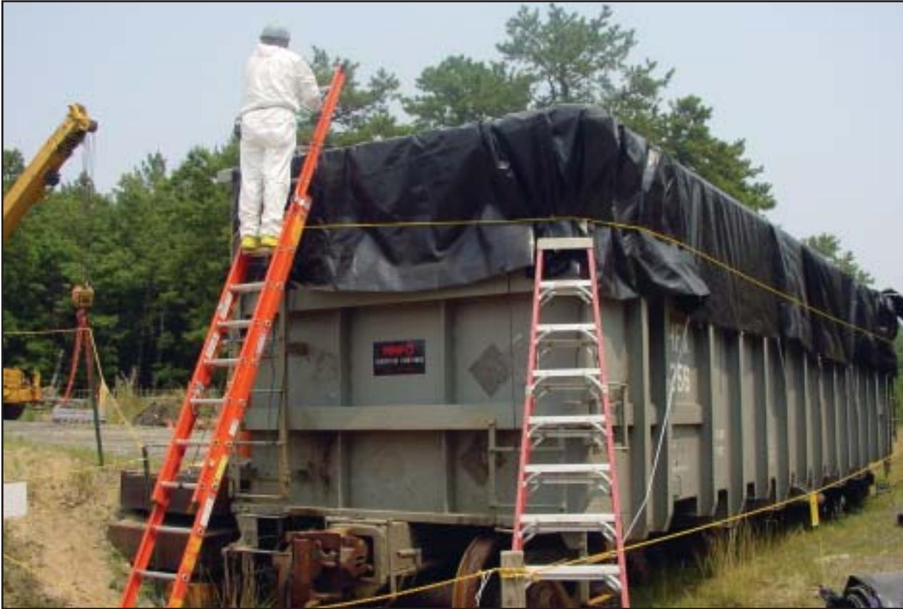
Worker installs Super Load Wrapper lining system in a gondola railcar prior to loading of low-level radioactive waste. Location: Brookhaven National Laboratory, Long Island, N.Y.
