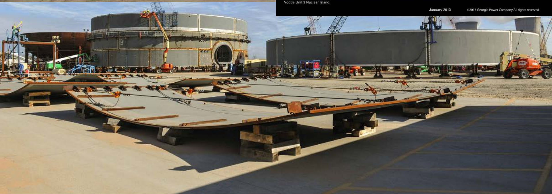
Assembly of Vogtle Unit 3 containment vessel rings (Unit 4 containment vessel bottom head at far left).
