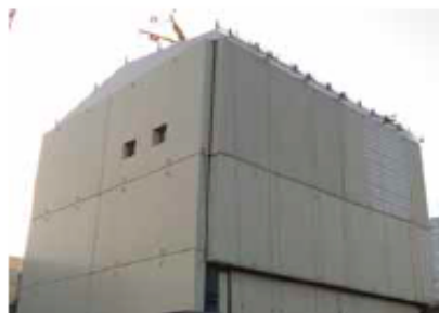
Unit 1 reactor building cover installation
