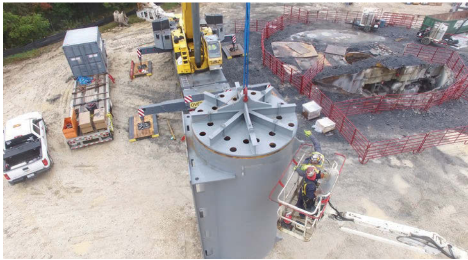
SEFOR, a site that pioneered research for reactivity control in fast neutron reactors, has been restored to its natural state. Shown is the removal and transport of underground reactor.
