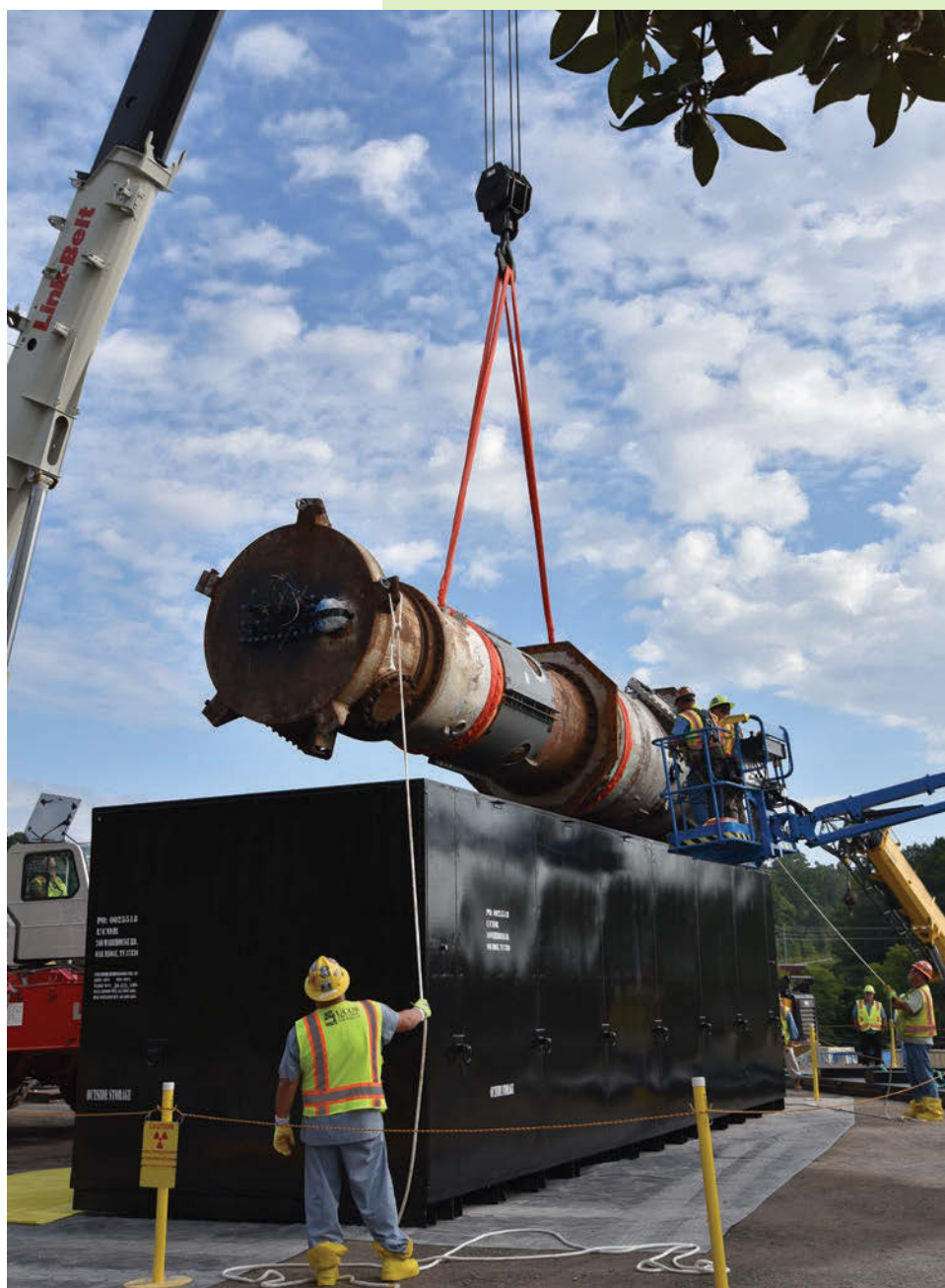
Reactor vessel from ORNL Low Intensity Test Reactor being lowered into its casing for transportation.
