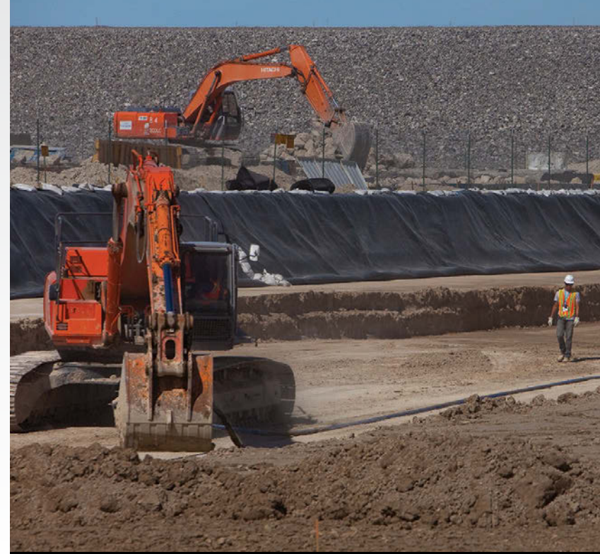
Clive Disposal Facility
