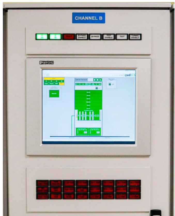
Operator-friendly visualization of diagnostic and process information ( typical HMI)
