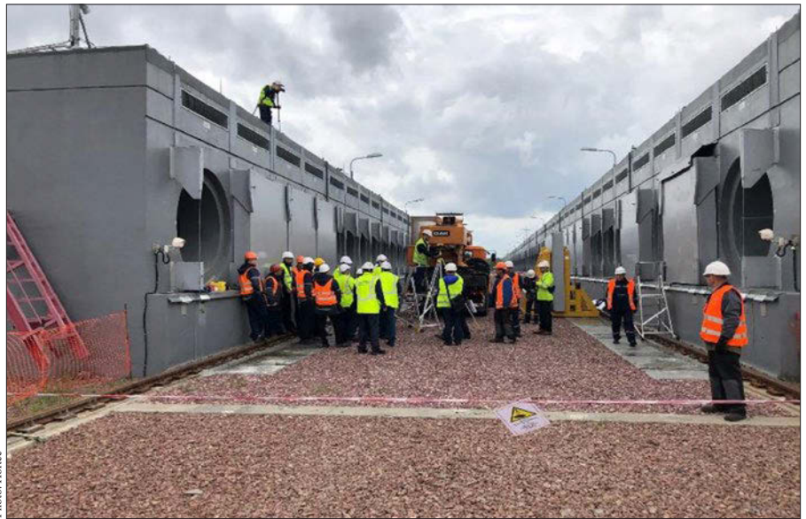
Workers conduct cold testing of the operability of Ukraine's ISF-2.
